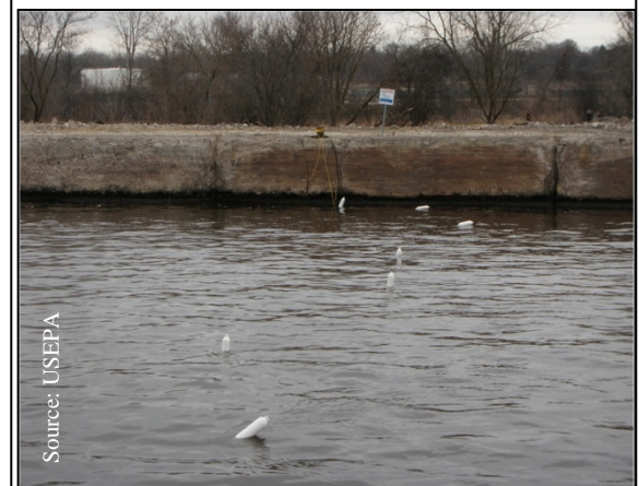
Buoys mark the location of submerged pipes across the CAWS for the rotenone
